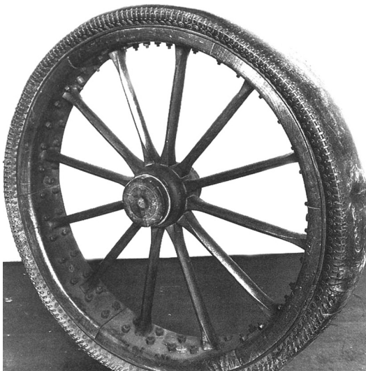
The Thomson pneumatic tyre as fitted to Loraine's Brougham in 1846
